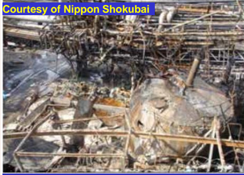
Photo 1: Destroyed AA Tank
